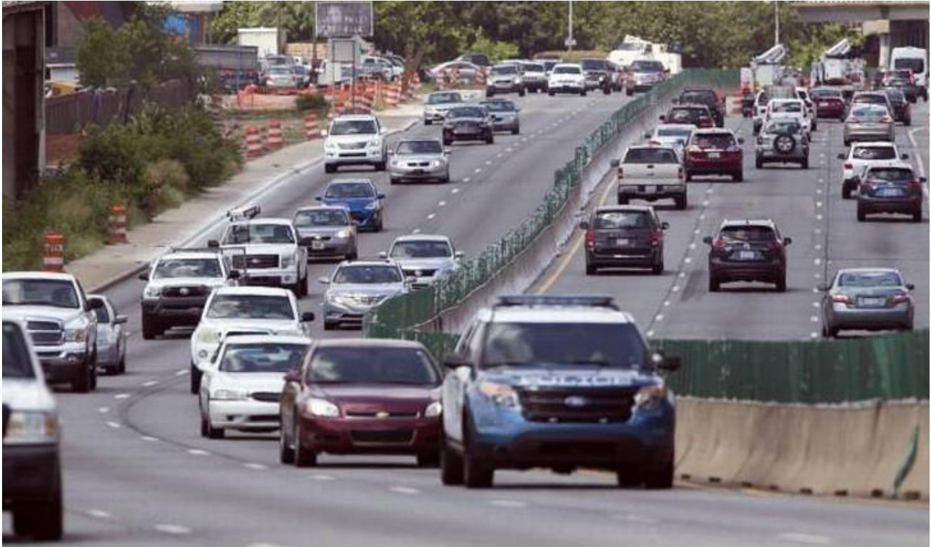
A congested corridor under construction- Robert Willett, newsobserver.com
